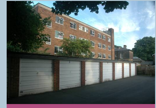
28. Rear extension to Highfield House
