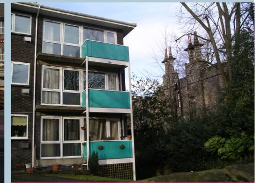
71. Inappropriate infill (North Hill Road)
