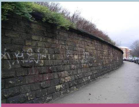
60. Reservoir Wall Clarendon Road
